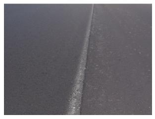
Figure 1.1-2 – Completed longitudinal joint with adhesive at Minnesota TH 100 during 2015 construction.
