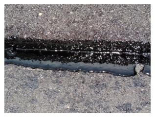
Figure 1.1-1 – Longitudinal joint with adhesive mastic at Minnesota TH 100 during 2015 construction.
